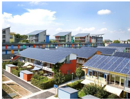
Figure 6 Roof-Top Solar Panel
